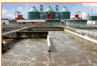
ETP / STP Plant Chemicals
